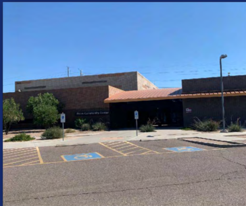
Ahwatukee Foothills Substation is situated nearby the Pecos Community Center
