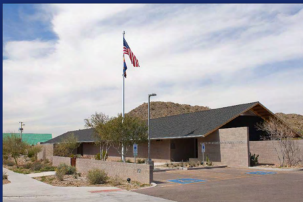
Sunnyslope Neighborhood Police Station
